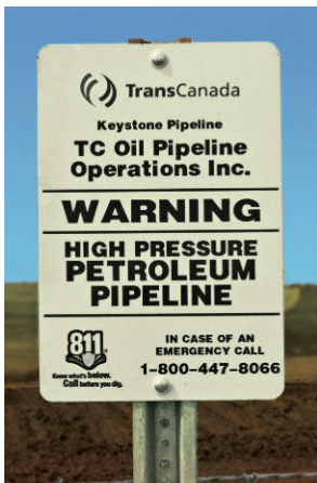
Typical TransCanada Keystone marker sign on the pipeline right of way (ROW) at road / railway and canal crossings
