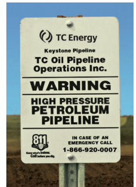
Typical TC Energy Keystone marker sign on the pipeline right of way (ROW) at road/railway and canal crossings
