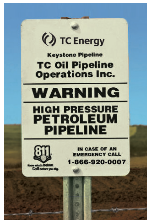
Typical TC Energy Keystone marker sign on the pipeline right of way (ROW) at road / railway and canal crossings
