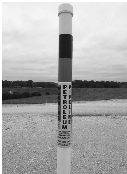
Our pipeline markers can be typically identified by the black and red bands at the top.
